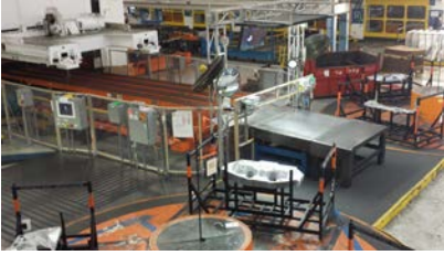
End of Line (EOL) System
